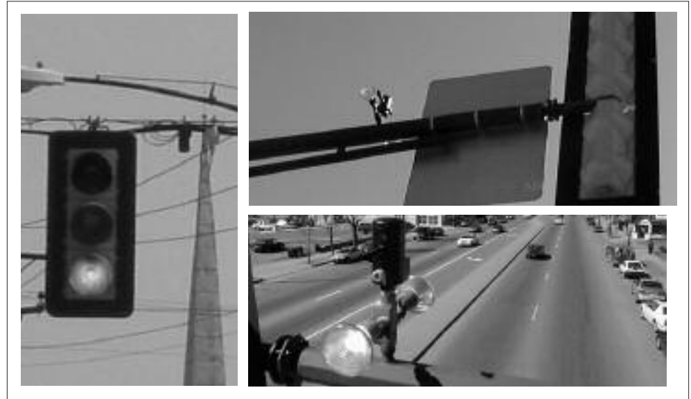
Figure 3 – Wire and Mast Arm Mounted Light-Based Detectors
